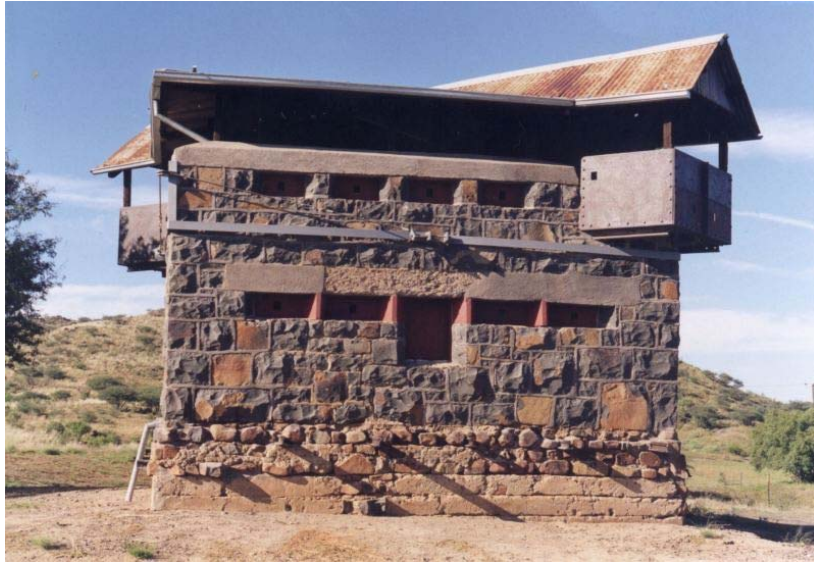
Orange River Station railway bridge blockhouse
